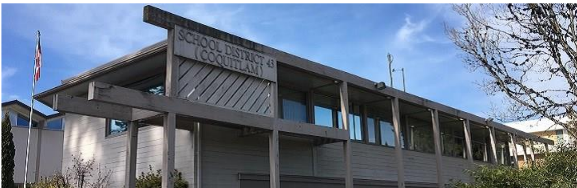
SD43's near 60-year old Board office is one of several aged-out buildings housing multiple administrative departments which would be relocated to the new ELC, along with other departments from other facilities.
